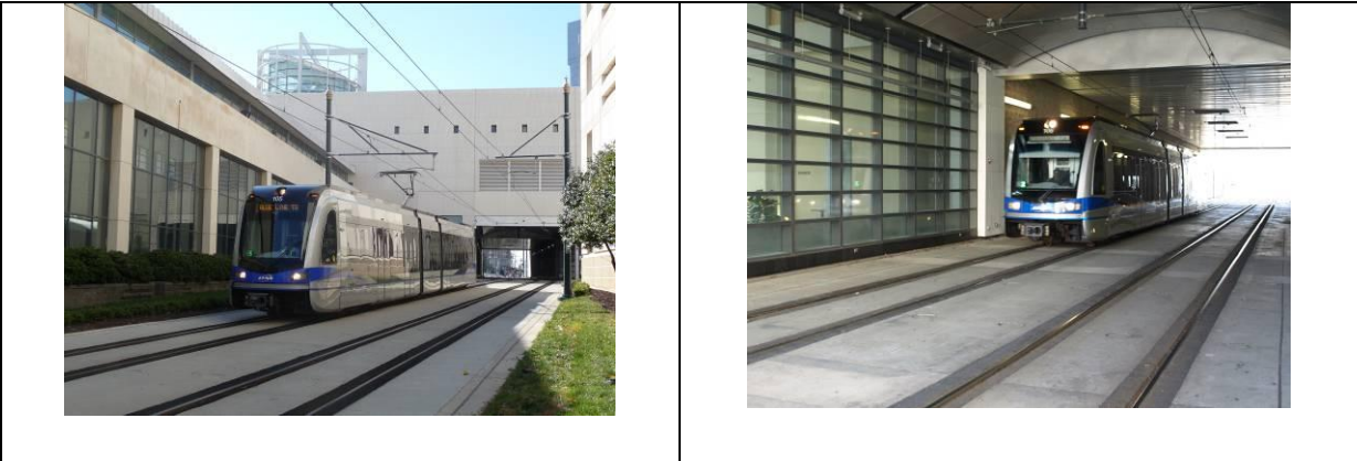
Figure 7: Tram passby through the convention center
